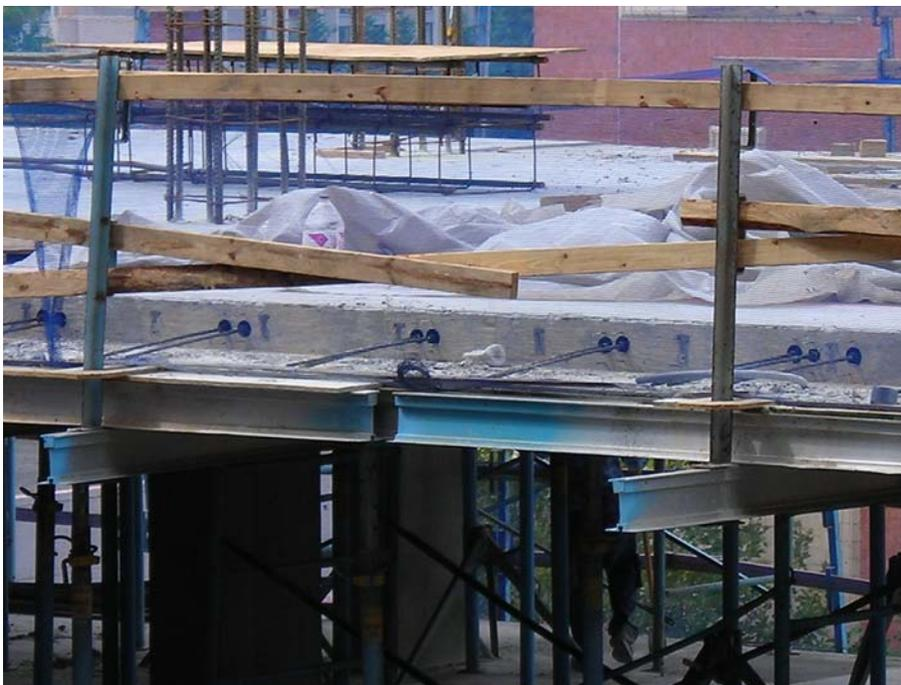
*Photo 10: View of post-tensioning cables prior to jacking force application.*
